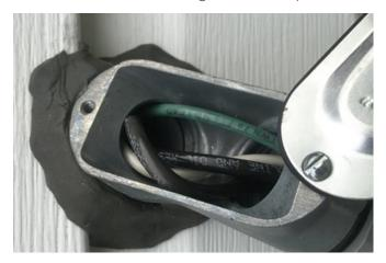
Photo 13: Two Hole conduit strap, with only one point of attachment, and no strain relief on conductors: NEC 110.3(B)
