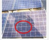
Photo 5 - Conductors over 30V not guarded, installed in raceway, or otherwise inaccessible: NEC 690.31(A)
