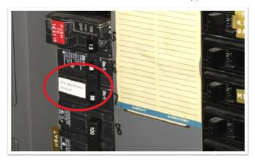
Photo 3: Working clearance not maintained: NEC 110.26
