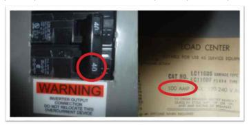
Photo 2: Backfed PV breaker not installed at opposite end of buss bar from main breaker: NEC 705.12(B)(3)(b)
