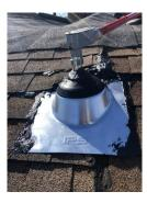
**Photo 7:** Where not protected from physical damage, equipment grounding conductor must be #6 or larger: NEC 690.46, 250.120(C). Conductors laying on asphalt shingles will become damaged and will not last a PV system's expected 30-year lifespan.
