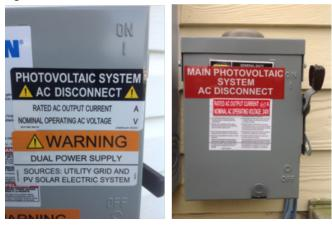
Make sure labels are permanent and suitable for use in the environment to which it will be exposed. In this example, these light duty adhesive labels will not withstand 20+ years of wind, sun and rain, and are in violation of NEC 110.21.
