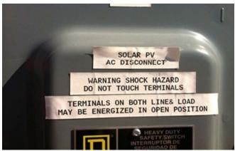
Label Not of Permanent Construction, nor conforming with NEC 690.31(G)(4).
