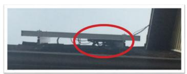
**Photo 9:** Equipment is not rated for location. In this case, a non-GFCI outlet for PV monitoring equipment is located in a wet location: NEC 110.3(B), 210.8(A)(3)
